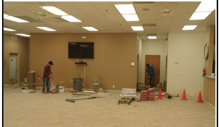
Workers completing the installment of the new tile flooring in our parish hall.
